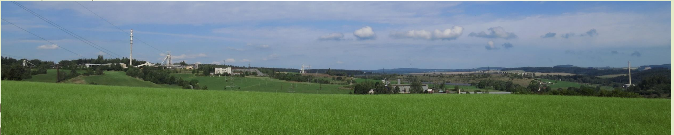
From left to right: chemical treatment plant, mine Rožná, mine Jasan, tailings pond K1 © Olga Kališová, Sept 2015
